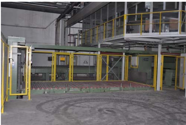
Extraction roller conveyor
